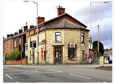
Walmersley Post Office
